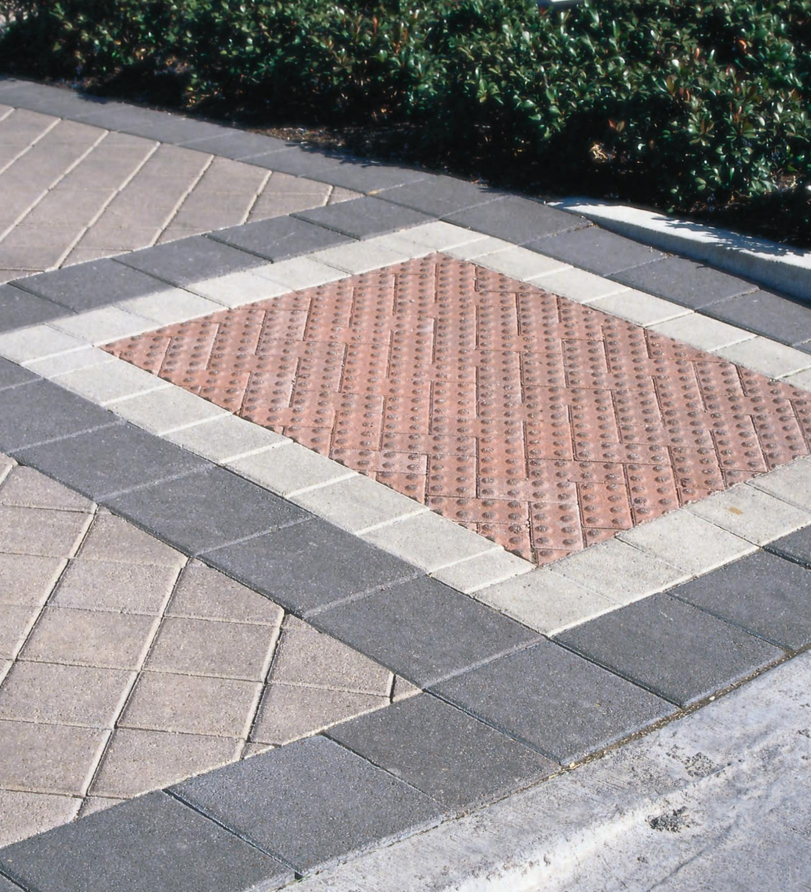
The ADA Detectable Warning paver provides visual and textural guidance provisions for wheelchair and pedestrian access to streets, sidewalks and other components of the public right of way.
